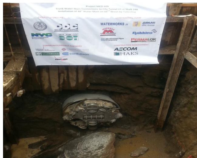
Micro Tunneling on West 62 nd Street
