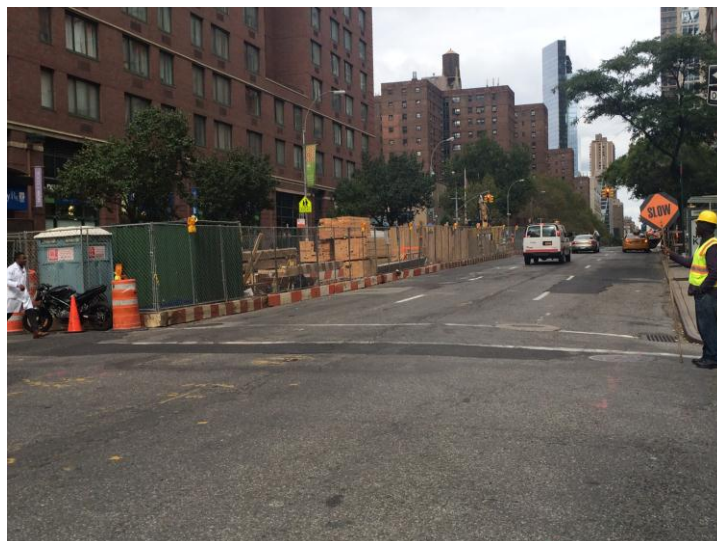
Excavation for 48" trunk main, looking north on Amsterdam Avenue from W. 59 th Street
