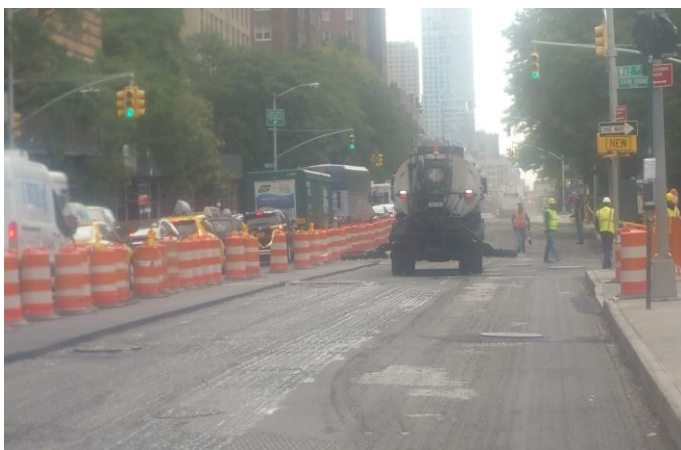
Final Restoration of Columbus Avenue from W.63 rd Street to W.60 th Street
