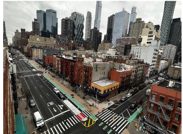
Modified Roadway Design of 9 th Avenue (NE view from W 52 nd St.)
